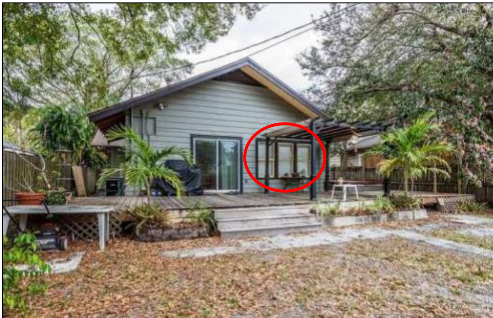
Figure 1: Photograph showing the windows to be removed.
