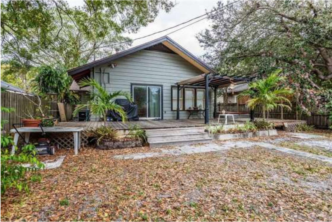
Back of house view showing 3 windows to be removed
